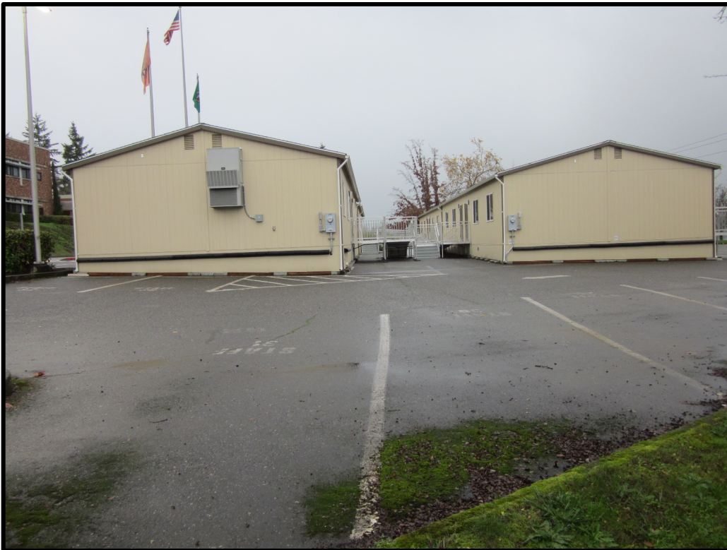
Figure 8. Typical conditions on the south side of the High School; view is to the east.
