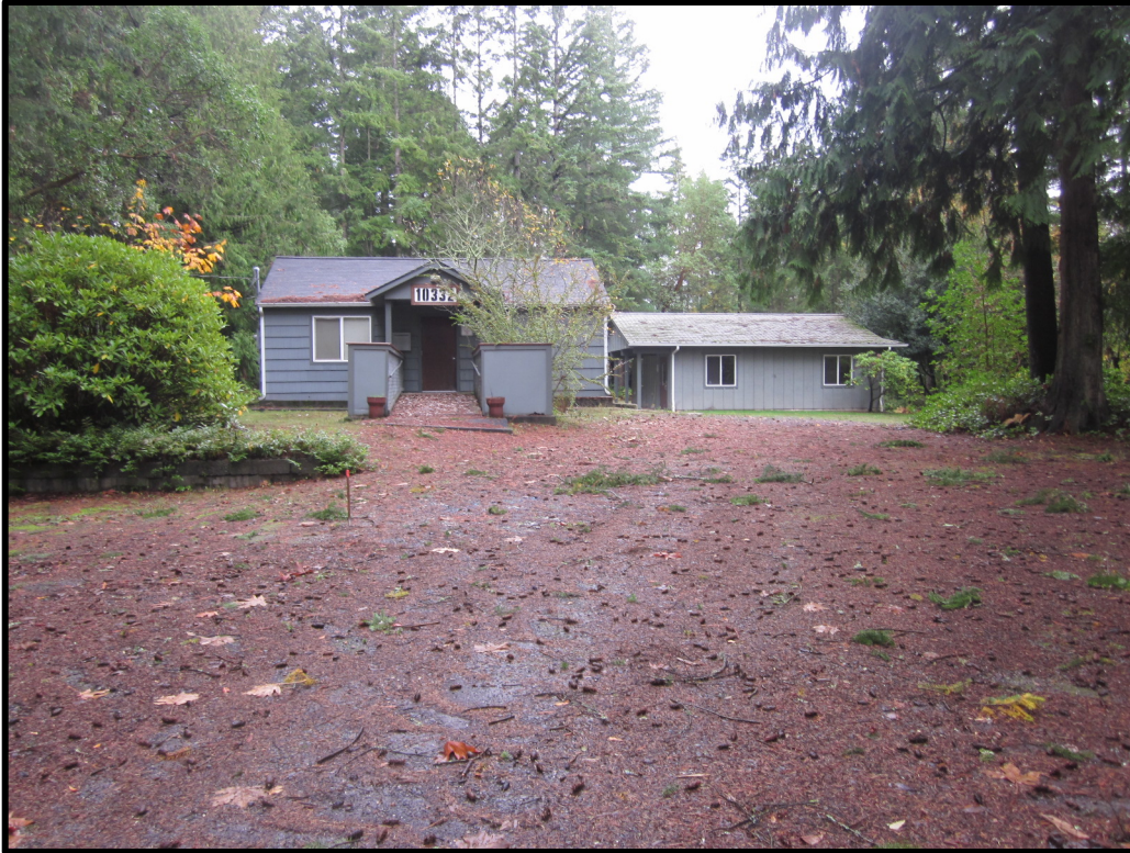
Figure 20. West elevation of former residence at 10332 Frontier Pl NW.
